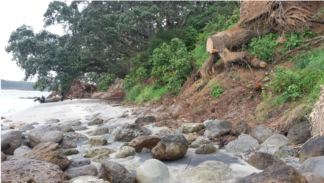
Photo 1 Soft sediment and hard shore/boulder marine habitats adjacent to slip area.
